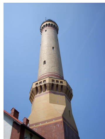
Fig. 7. Świnoujście lighthouse – contemporary view.
