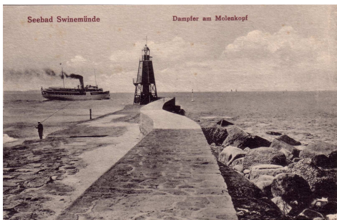
Fig. 6. Entrance beacon (3) on eastern breakwater
